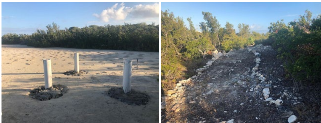
Figure 4. Clearance of trail and preparation for viewing hide at Wheeland Pond
